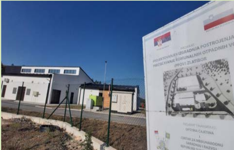
there are no mentions of the EU on-site observations, Wastewater treatment plant of Zlatibor - Entrance, August 2023
